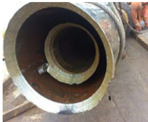
The 20 inch x 35 inch Cut Casings
